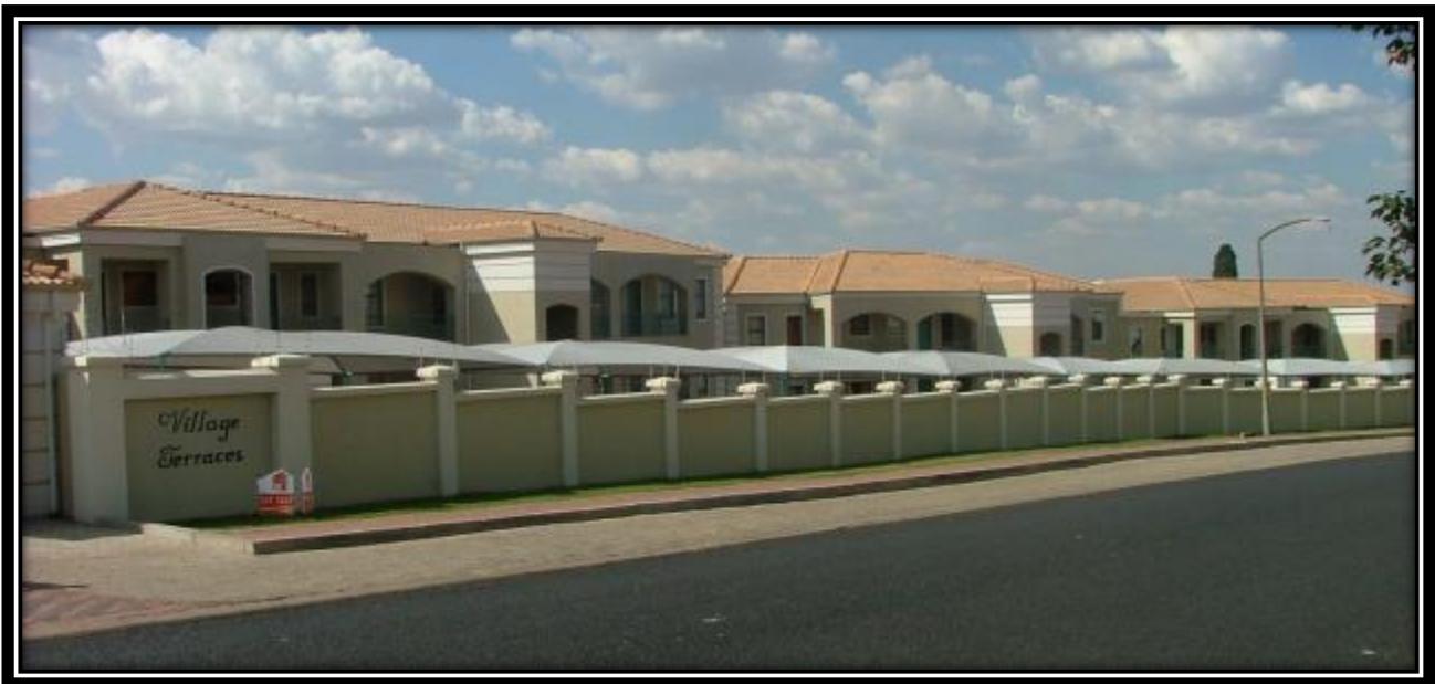
28 units @ Village Terraces
